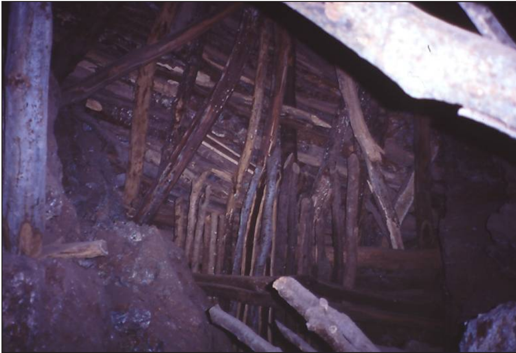
Photo 5 Timber wall holding up backfill, Socavon Intermedio (McBride Photo)
